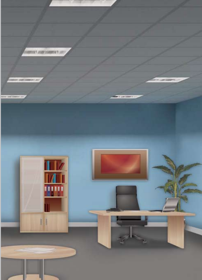
Depressing and uninteresting: Traditional recessed louvre luminaires alone create a gloomy office with the 'cave effect'
